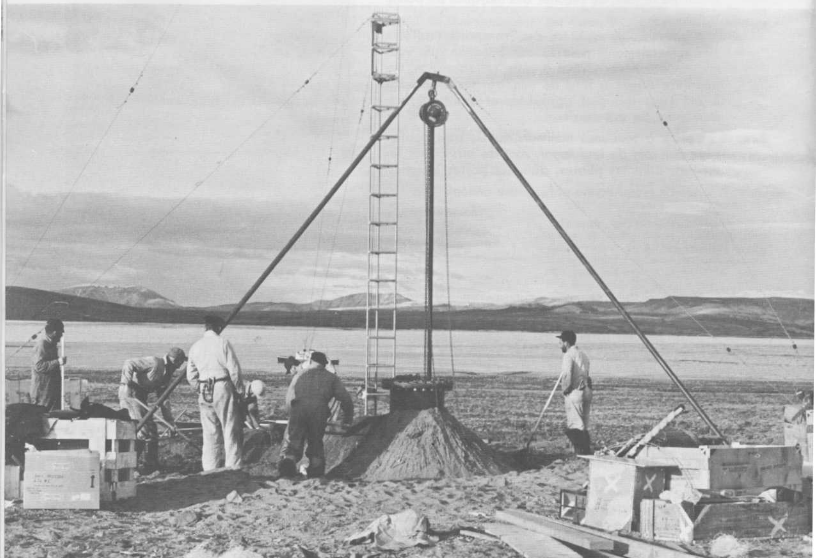
ARCTIC WEATHER EYE —Volunteer workers from CMS John A. Macdonald help with installation of world's first isotope-powered automatic weather station. Steel cylinder (centre) containing electronic deck and isotope unit is partially buried in permafrost on Axel Heiberg Island in High Arctic. Icebreaker is seen in background.
