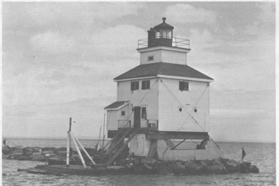
It's a good life, the men who man our lighthouses that dot the islands and coastline of rugged Lake Superior will tell you. Above is the main lighthouse at the entrance to the harbour at Port Arthur, Ont.
