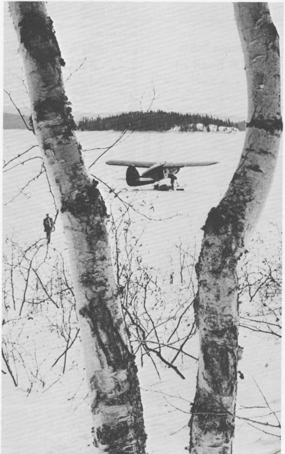
Main route to the north.
