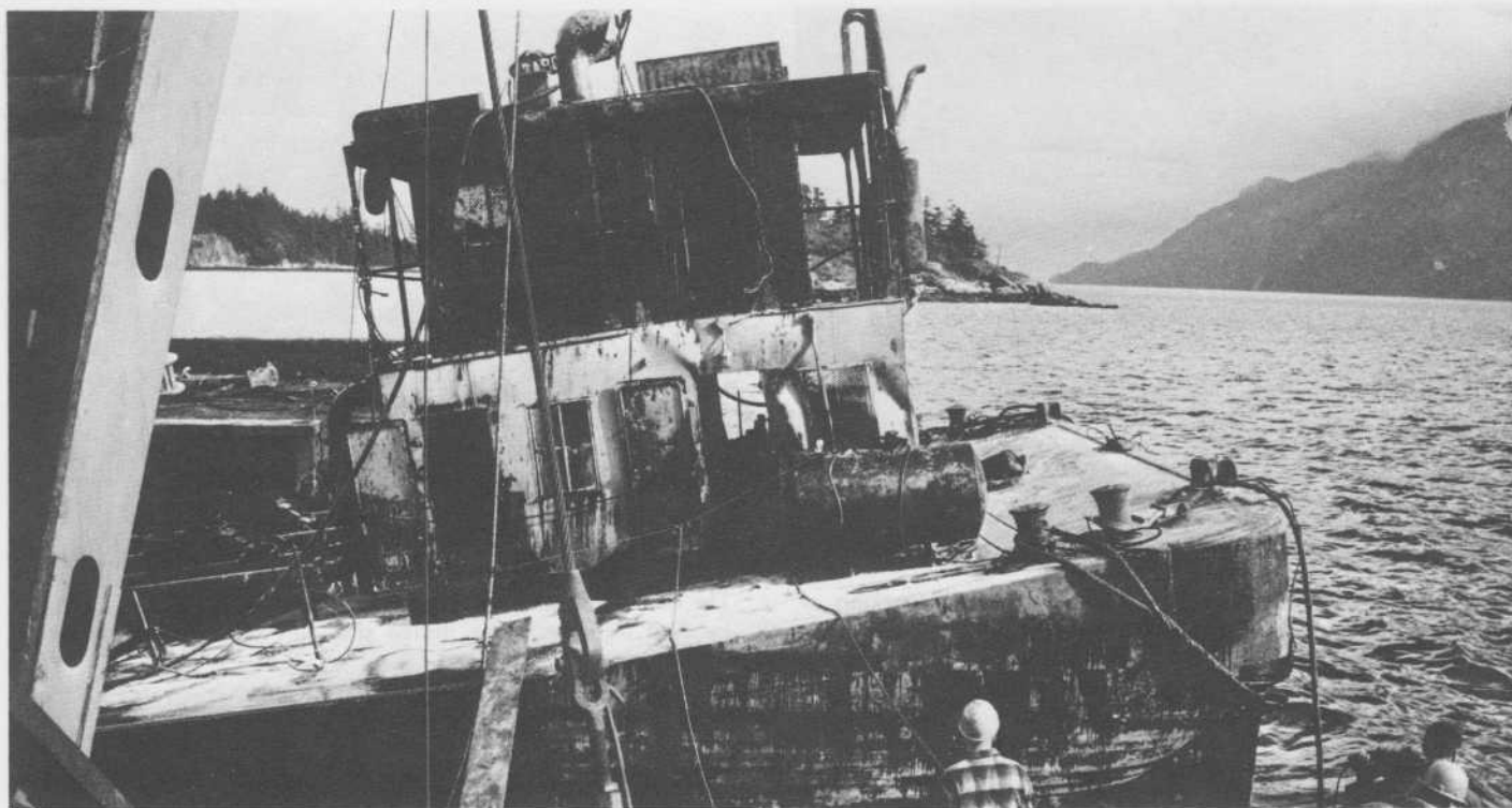
Stern of oil-blackened barge as it was being brought to surface. At this point the bow was still resting on bottom in 28 feet of water.
