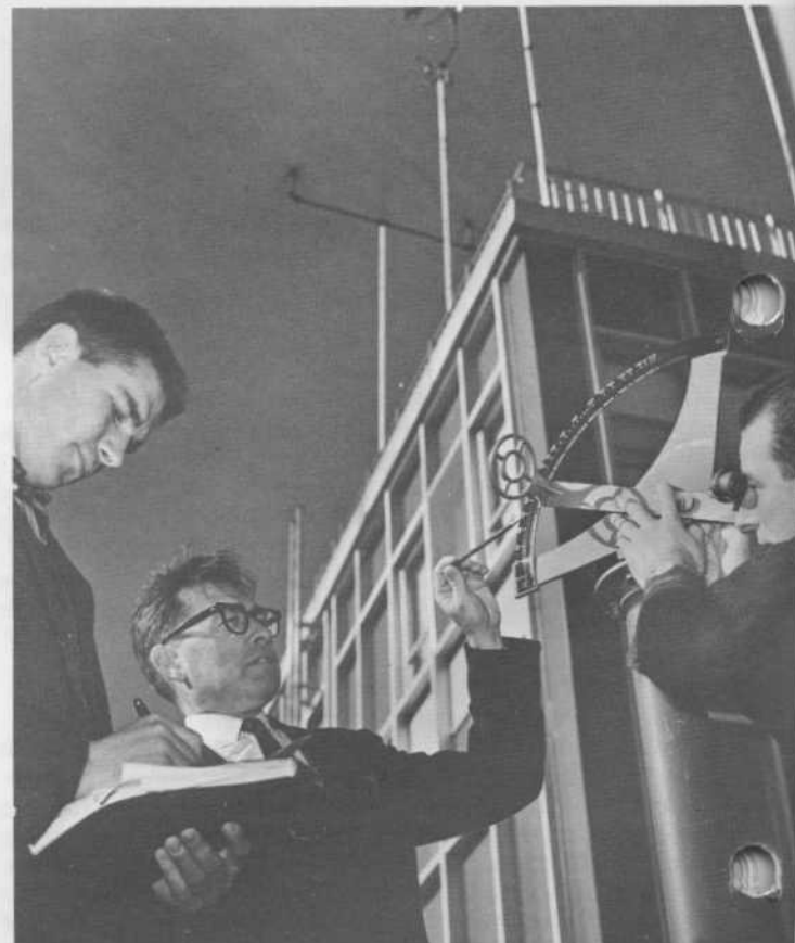
WEATHER-WISE —Student weather observers take readings on roof of terminal building.
