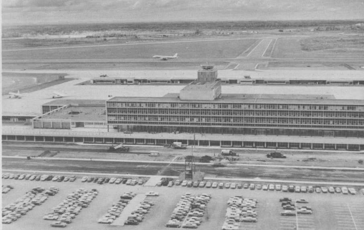
Aerial photo shows ramp by which departing travellers arrive at building. Parking lot accommodates 1,500 cars. Aeroquay behind building serves all overseas and all jet flights.
