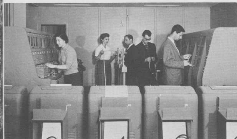
Marine-aeradio tape relay centre in terminal converts typewritten messages into punched tape for fast relay. Communicators, from left: Miss L. Bedard, Miss E. Neville, Y. Clement, J. Ouellet, J. M. Paquin.
