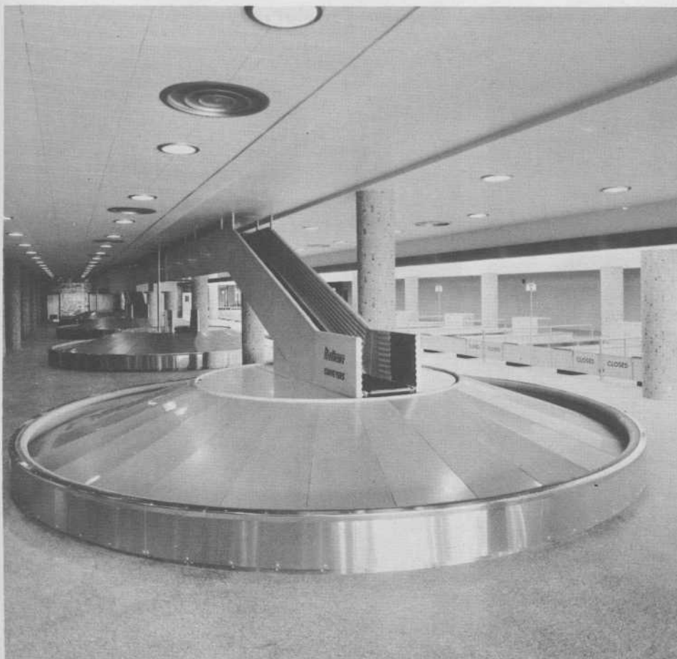
Rotating baggage dispensers speed up luggage handling in international section. Similar conveyors serve domestic travellers. At right is long line of customs counters designed to minimize delay.
